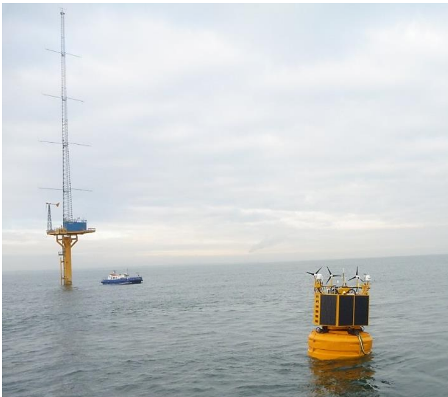
Figure 4-4 FLiDAR nv deployed for validation at Blyth
