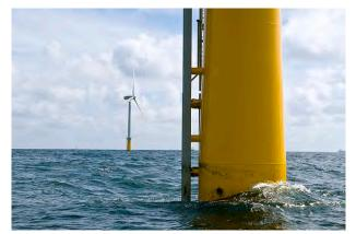
Figure 2.3 Examples of Mono-pile Foundations (a single pile into the seabed) (Source: https://commons.wikimedia.org/wiki/File:Prinses Amalia Windpark.jpg)
