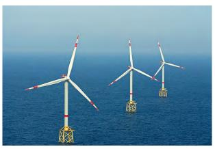
Figure 2.4 Examples of Turbines on a Jacket Structure
