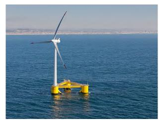
Figure 2.5 Example of Floating Wind Turbine - Windfloat by Principle Power (© Principle Power Inc/licence details: <u>https://commons.wikimedia.org/wiki/File:Agucadoura\_WindFloat\_Prototype.jpg</u>)
