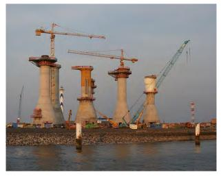
Figure 2.2 Example Concrete Gravity Foundations/Structures – Thornton Bank project (© Hans Hillewaert/licence details: <u>https://commons.wikimedia.org/wiki/File:Windmill\_bases\_(Oostende - from\_northwest).jpg</u>)
